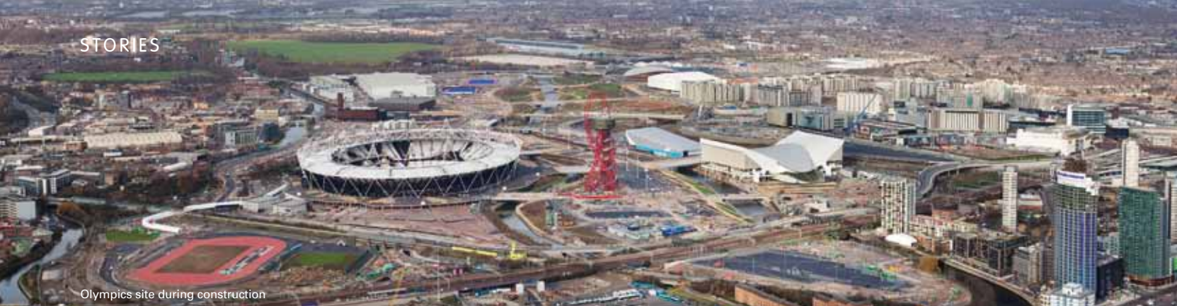
Olympics site during construction
